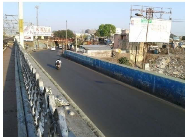
Fig. 1(b) – Road Bridge close to Railway track
